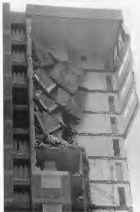
Plate No 2 Close-up of damage showing wall . . . streaming backwards and forwards like a flag . . .
